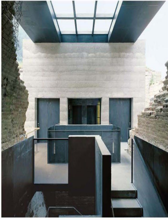
The stair and elevator entrances are contained in a small concrete-and-steel building. Pumpkiner Area Rider
