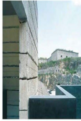
Like the last shell, the intervention consists of simple materials: concrete and black-painted steel. Pumpkiner Area Rider
